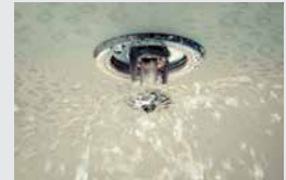
Broken Sprinkler
