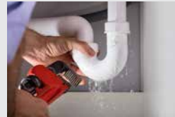
Burst Water Pipe
