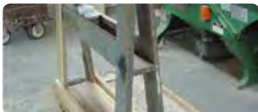
Wood - Splinters and rots
